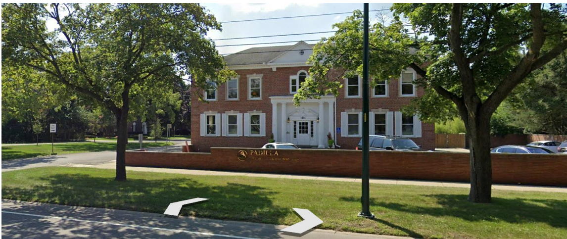
Figure 18: Above, Existing 12,000 sq. ft. office building, W. Maple-Larchlea Streets.
