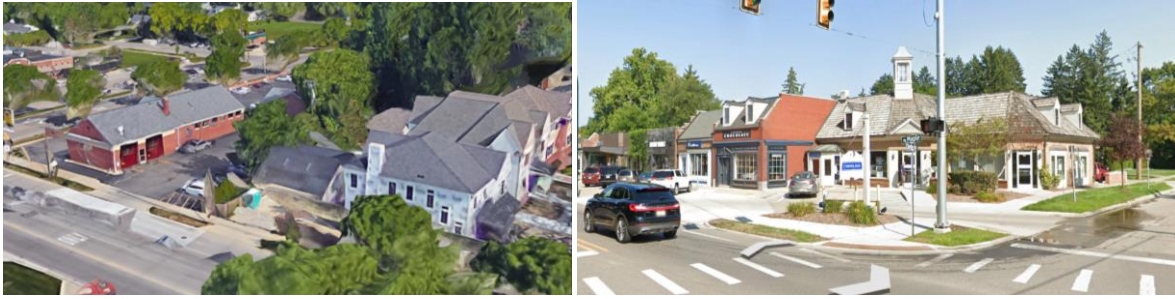
Figure 2: Above left, new house construction behind an auto service center, 14 Mile and Southfield Streets. Right, view of the Quarton Lake neighborhood's 20,000 sq. ft. shopping center: Chester and W. Maple Streets. Note, the center's corner bank building originally operated as a Mobil gas station.
