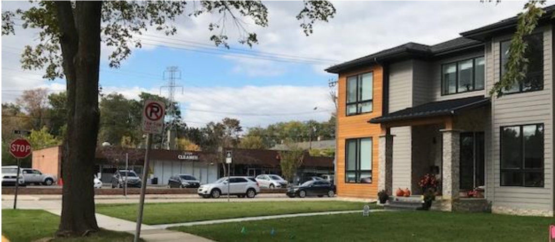
Figure 17: Yorkshire Street looking west towards N. Eton Street towards 2 neighborhood shopping centers. The commercial buildings total 12,000 sq. ft. and include a café, cleaners, food market, hair salon, seamstress and carry-out pizza restaurant.
